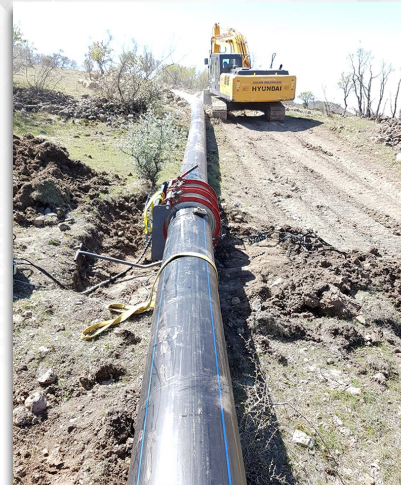
Image-1: Welding the pipes arranged on the trench route to each other with Butt Welding.
