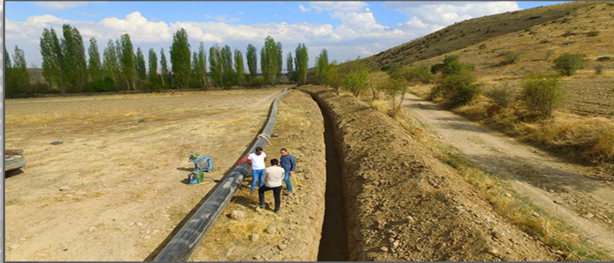
Image-2: Arrangement and welding of pipes on the edge of excavated trench
