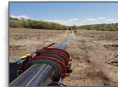
Image -7,8,9: Installation and fixing of pipes in welding machine
