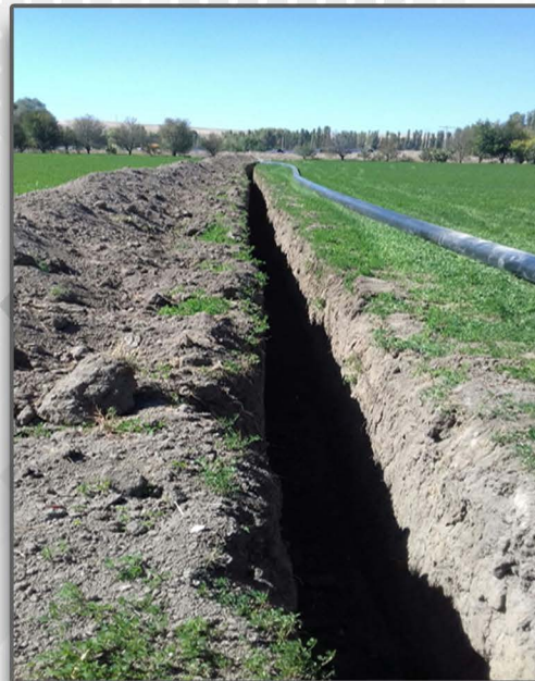
Image-3,4,5: Trench Excavation
