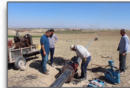
Image -7,8,9: Installation and fixing of pipes in welding machine
