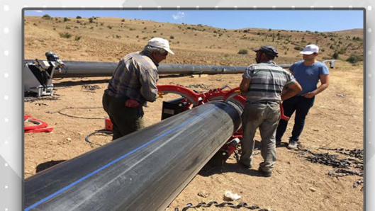
Image -7,8,9: Installation and fixing of pipes in welding machine
